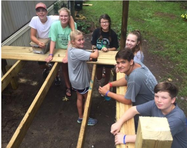
Picture at the beginning of the project completed
